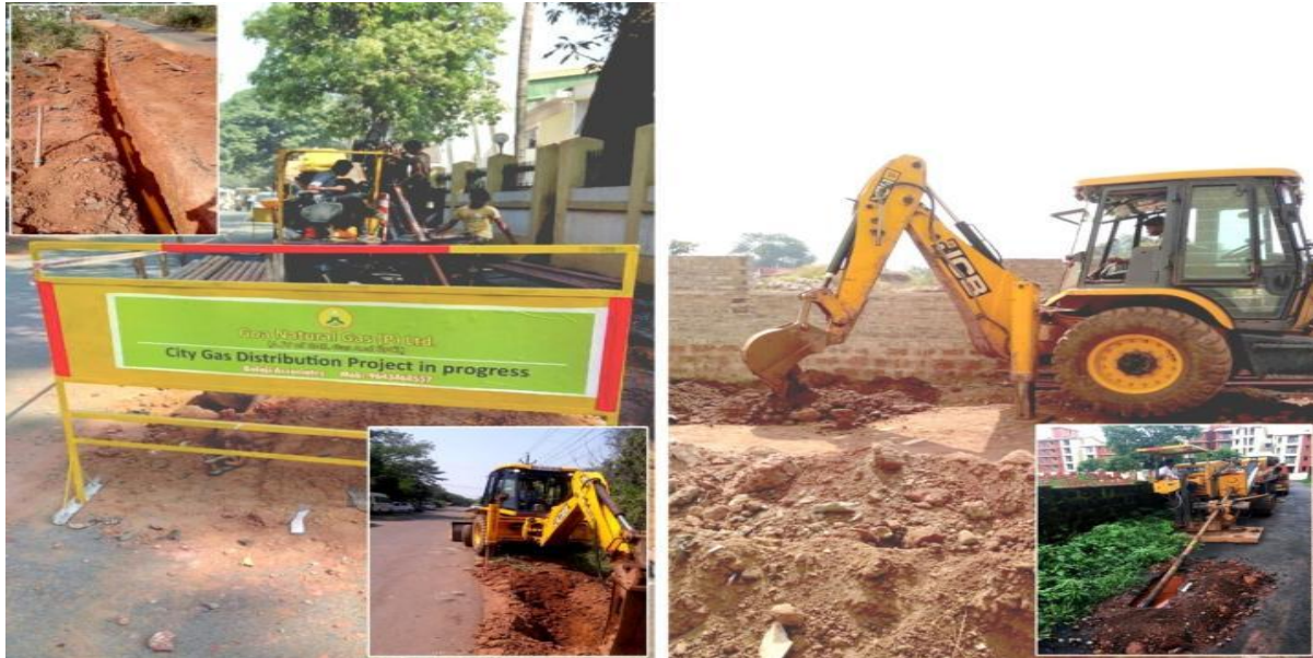
MDPE Pipe laying in progress.....
