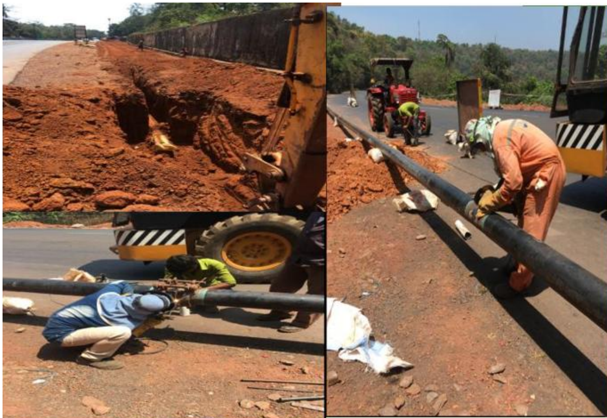
STEEL Pipe laying in progress.....
